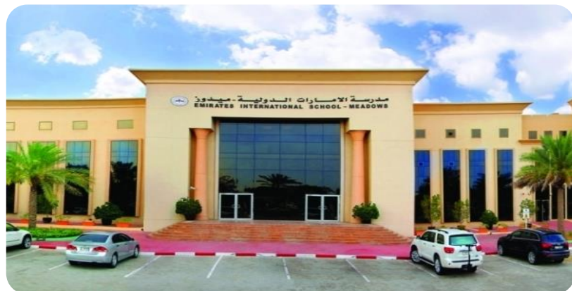
Emirates International School Expansion - Dubai
