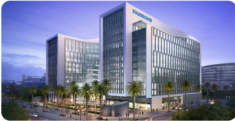
Parsons Head Quarters Abu Dhabi
