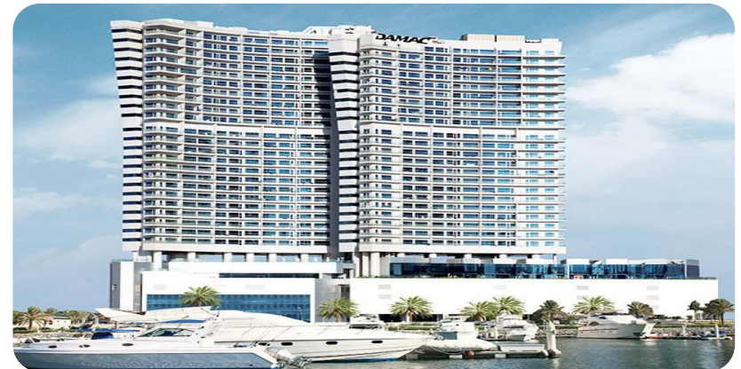
DAMAC Oceanscape - Mixed Use DAMAC Complex, Al Reem Island
